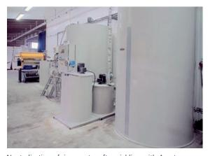
Neutralisation of rinse water after pickling with Avesta-BML Neutralising Facility.
