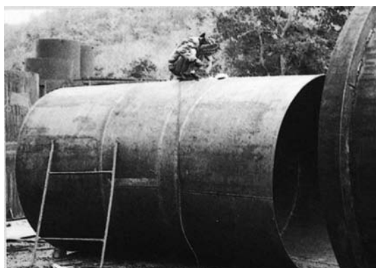
Water tanks with a thin section are often fabricated with RB-26 in Thailand.
