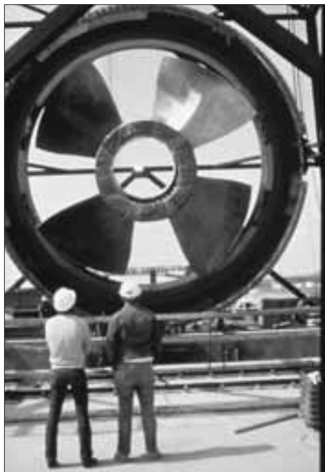
Figure 1.5. Hydro electric power turbine in 248 SV
